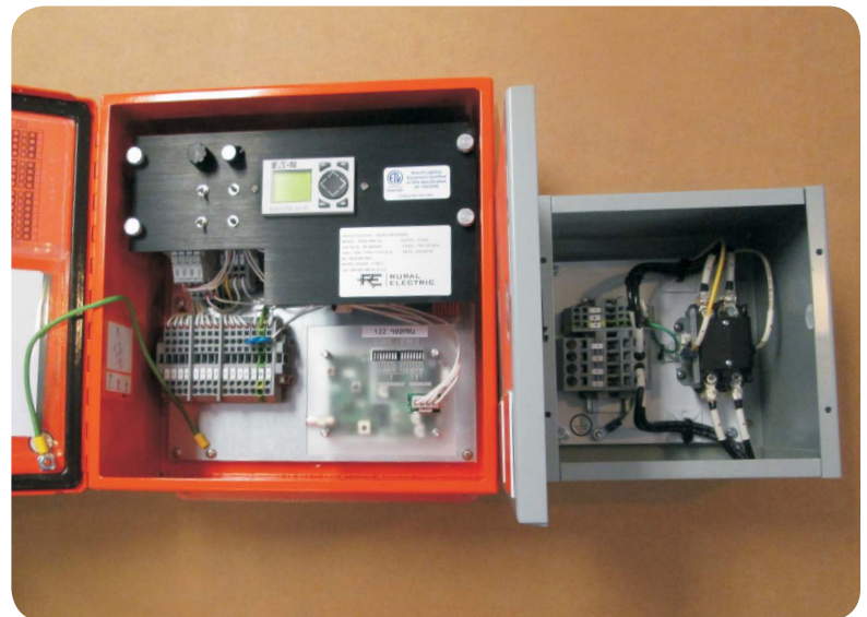
Heliport Control Box shown with L-854 Controller
